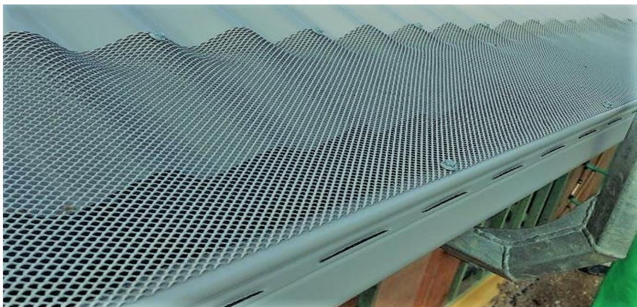
Figure 1.2 - Standard GPS Ember Guard installed on Corrugated roof without Water Brake.
