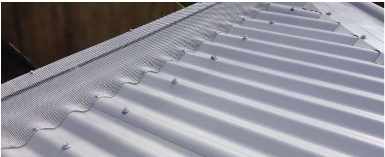
Figure 1.3 - GPS Ember Guard, a non-combustible gutter fitting.
